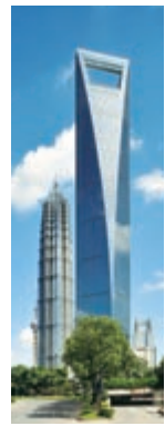
Elevators for the highest building in China (Shanghai World Financial Center)
