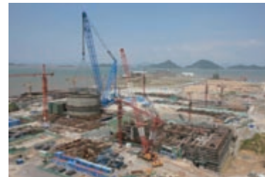
Construction of the Sanmen Nuclear Power Station in Zhejiang Province, China
