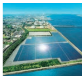
(Artist's rendition) Chubu Electric Power Company's Taketoyo Mega Solar Power Plant
