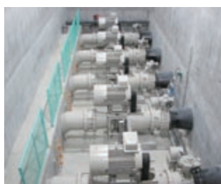
Mibugawa No. 4 Plant, Mibugawa Electric Power Co., Inc.
