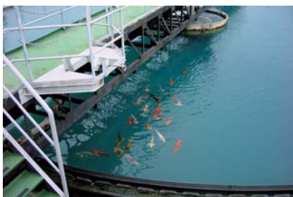
Wastewater treatment facility
