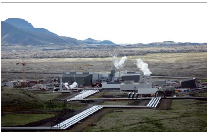
Hellisheidi power plant (in Iceland)
